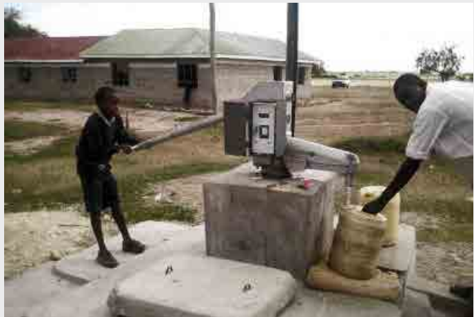
A community water point with a pre-paid meter that enables users to pay a small amount of money to take care of operations and maintenance. | Photo credit: Maji Milele
